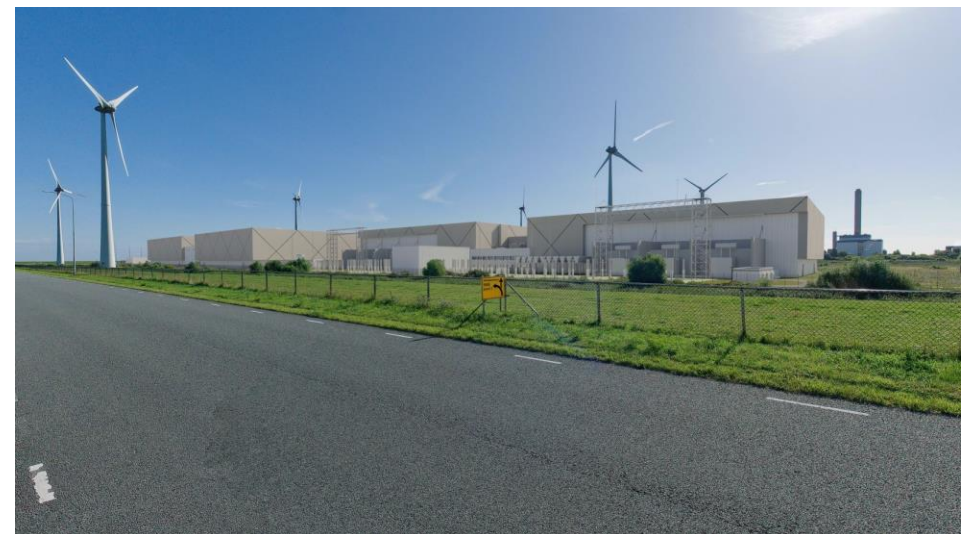
Two converter stations in Eemshaven
